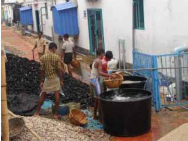
Preparation of sand filter
